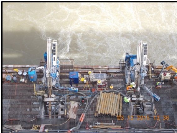
Drilling using Modified Platform Configuration
