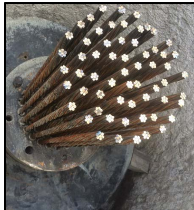
High Capacity, Multi-Strand Anchor Installation
